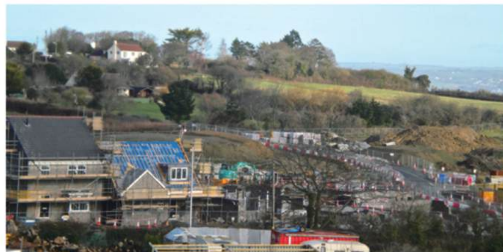
Wooda Road development looking towards Appledore.
