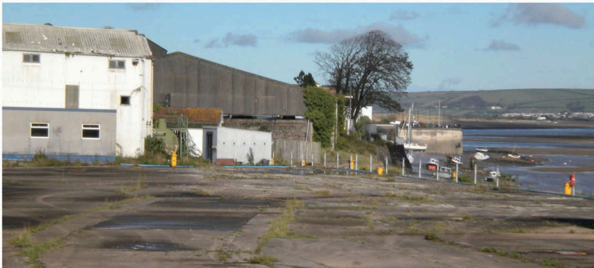
Site of New Quay Dry Dock, Appledore
