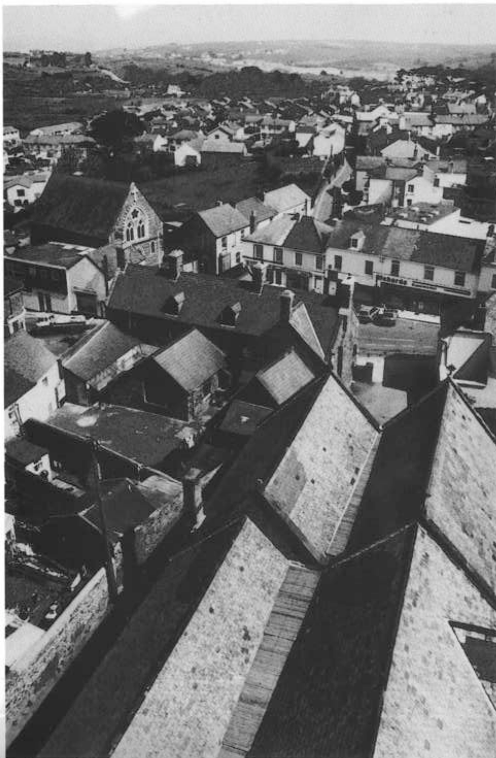
View from the top of St. Margaret's Church tower towards the River Torridge.
