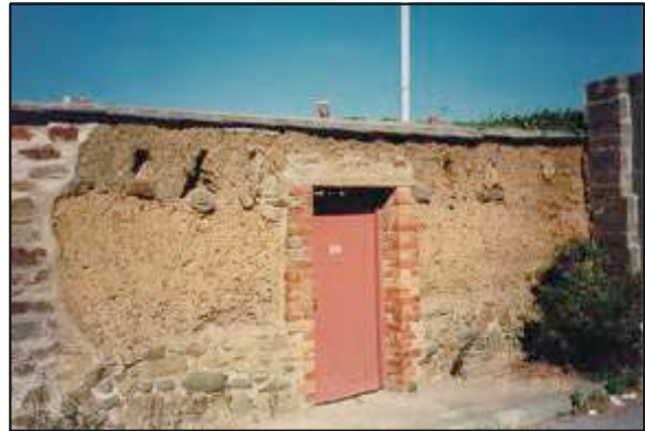
Cob walling, rear of Irsha
